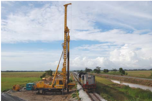
Fig. 22 Installation of Stone Columns adjacent to Existing Live Track.
