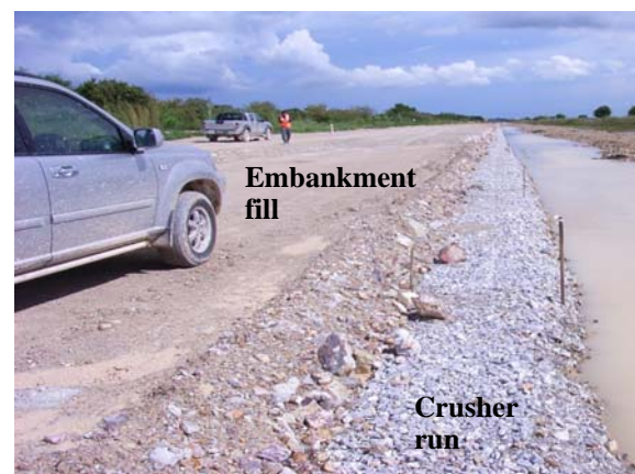
Fig. 19 Details of Discharge Outlet for Sand Blanket Connecting All PVD
