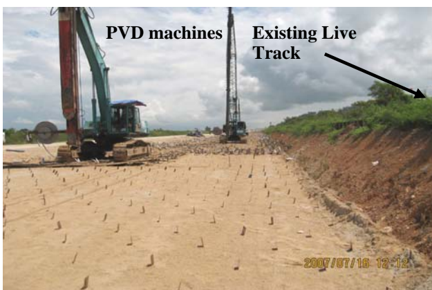
Fig 20 Typical PVD Machine working beside the Live Track
