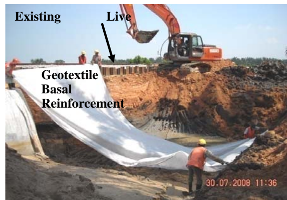
Fig.21 Typical Cross Section and photo showing Geotextile Basal Reinforcement
