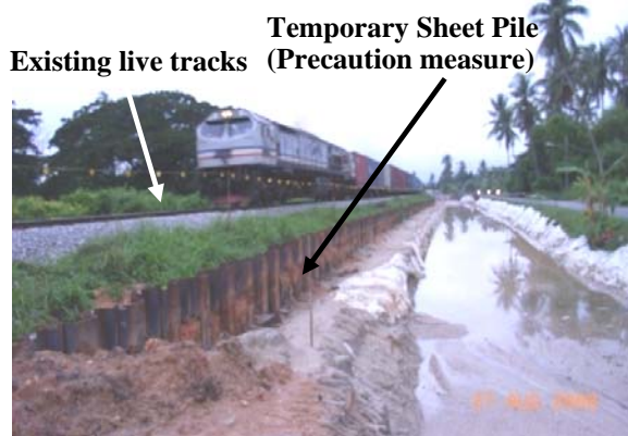
Fig. 15 Typical Cross Section and Photo showing Temporary Sheet Pile for E&R.
