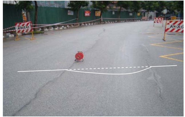
Fig. 10. Subsidence trough developed on the retained ground.
