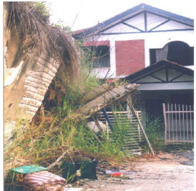
Figure 14: Failed RC Wall
