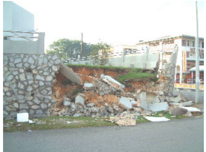
Figure 13: Collapsed Rubble Wall
