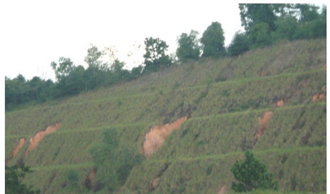
Figure 12: Localised Erosion on Slopes
