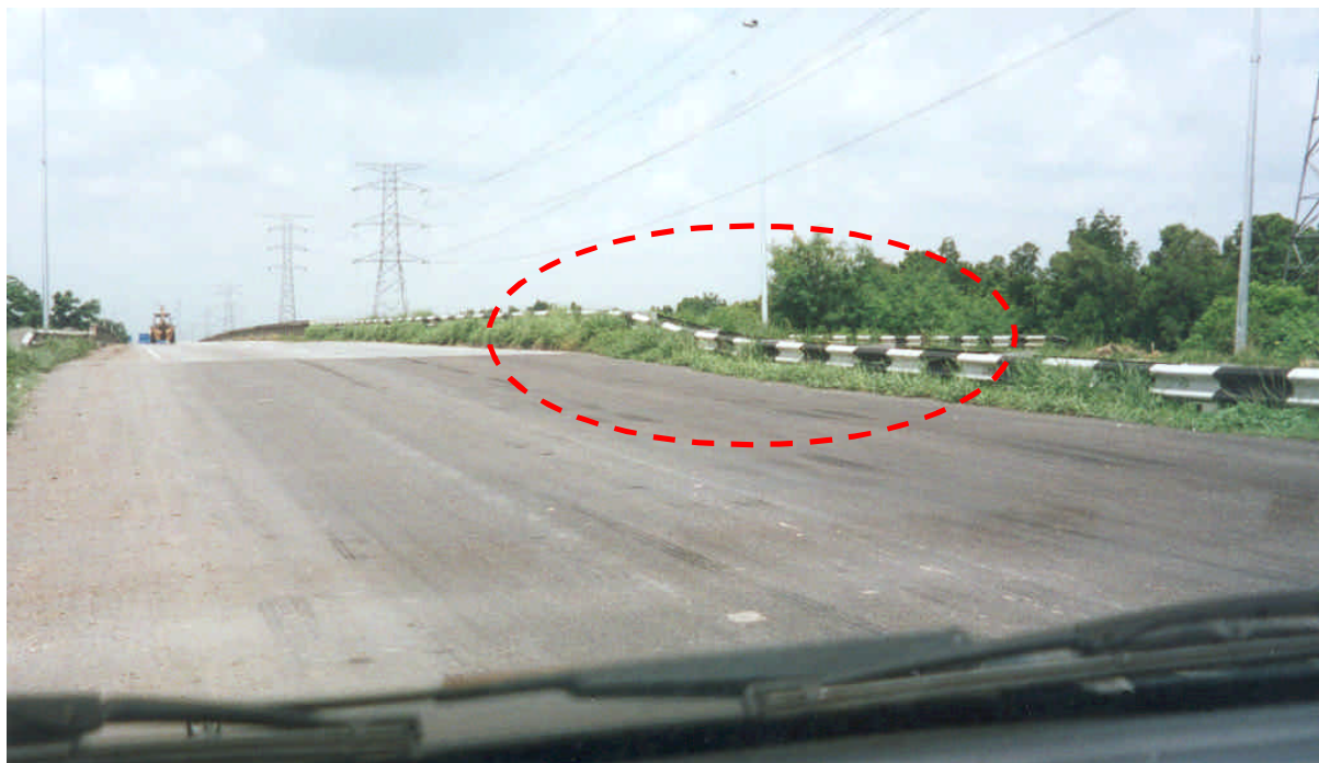
Plate 2: Hump at Bridge Approach
