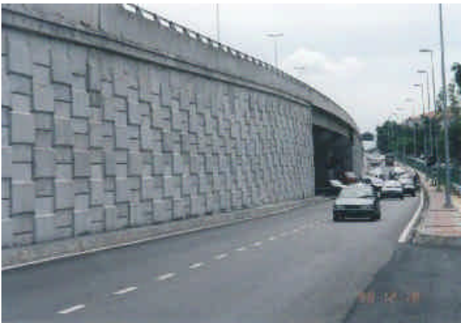
Photo 1: Side View of the RE Wall Embankment
