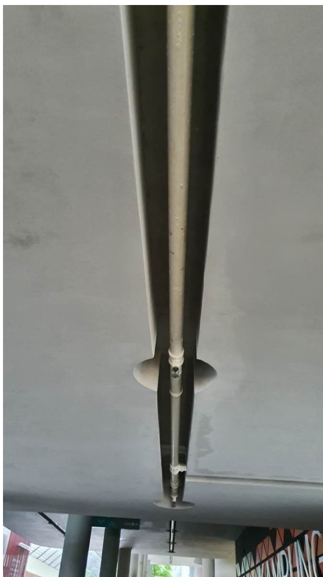
Figure 2 : Engrooved Springer System into Precast Slab
