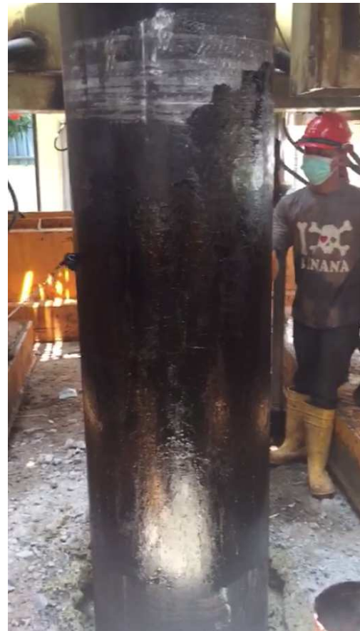
Figure 4 Application of Bitumen with Primer Coating as Debonding Material during Pile Installation
