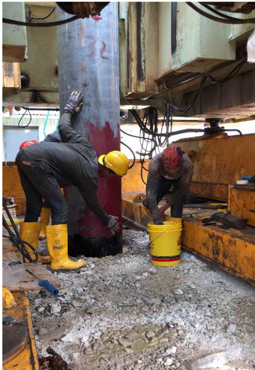
Figure 2 Application of Heavy-Duty Mechanical Grease as Debonding Material during Pile Installation
