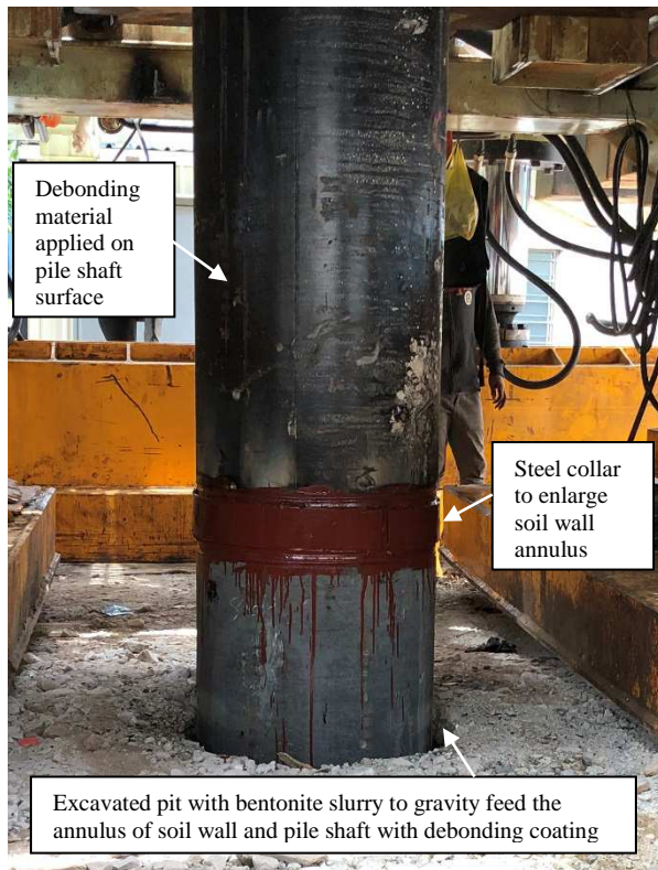
Figure 5 Primer Coat as Debonding Material
