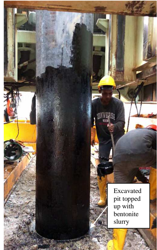
Figure 3 Application of Bitumen as Debonding Material during Pile Installation
