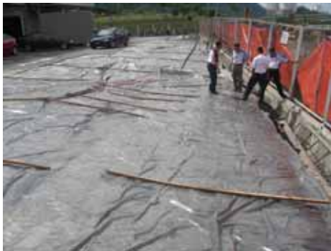
Ground Distress at Active Wedge
