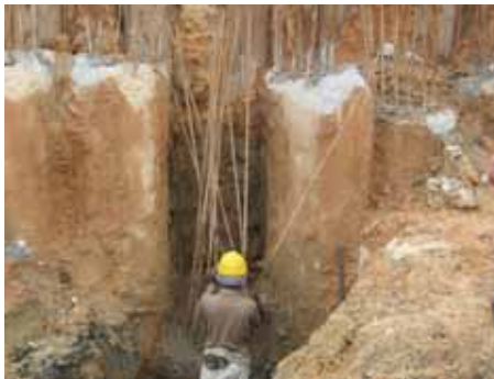
Repairing of CBP Pile
