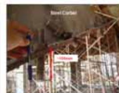
Post-installed Bolts After Wall Failure
