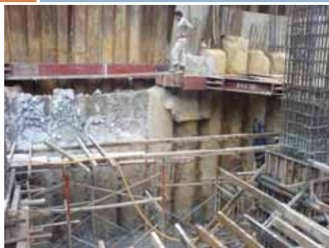
Repairing Crushed CBP
