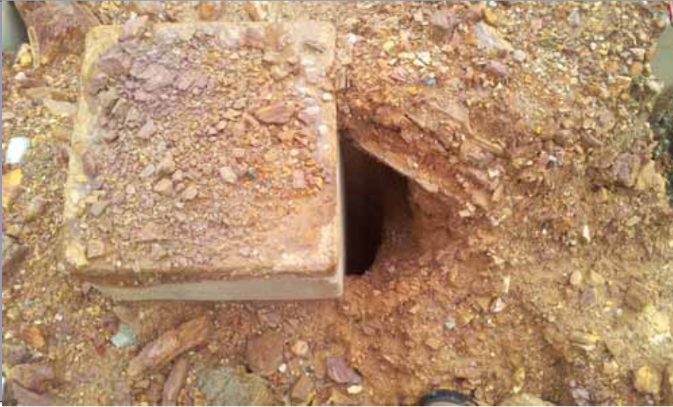
Void in Pre-bored Hole Annulus
