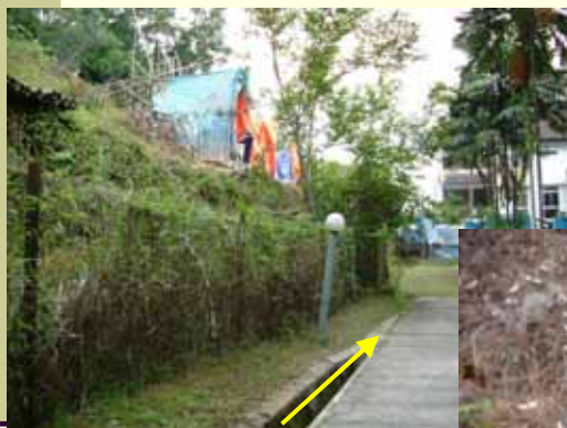
Closed Drain at Toe of Slope
