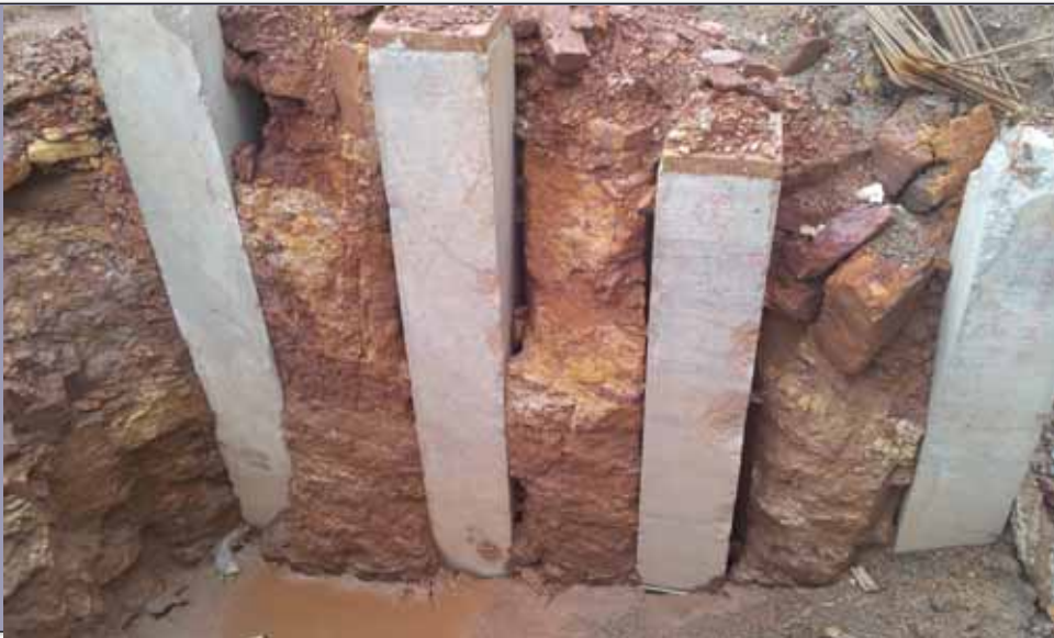
Collapsed Debris in Pre-bored Hole Annulus
