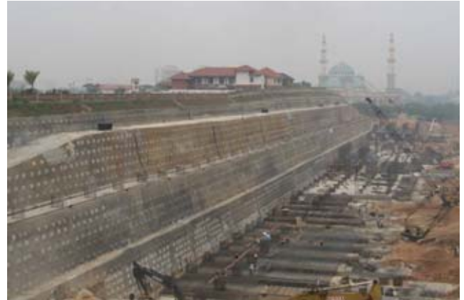
Figure 3. 30m high soil nail slope.
