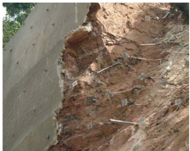
Figure 4. Example of face failure.
