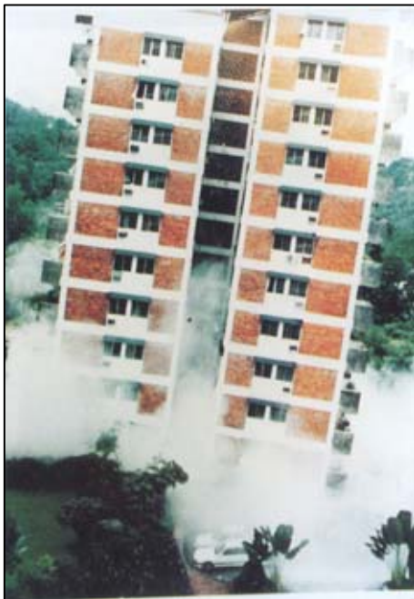
Figure 1 : Block 1 Starts to Topple (from MPAJ, 1994)
