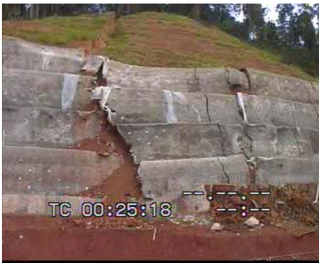
Figure 5. Front view of failed soil nail slope.
