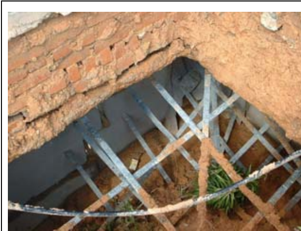
Figure 4 Voids Behind Wall Due to Backfill Materials Being Washed Away
