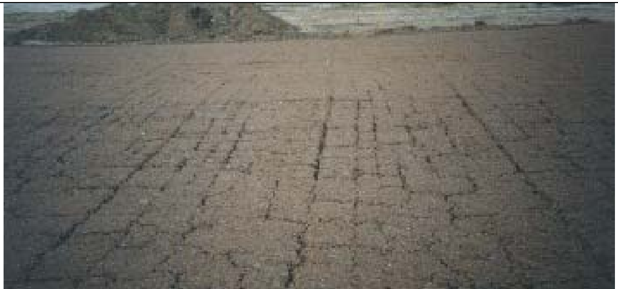
Figure 12 Shrinkage Cracks at Runway Subgrade
