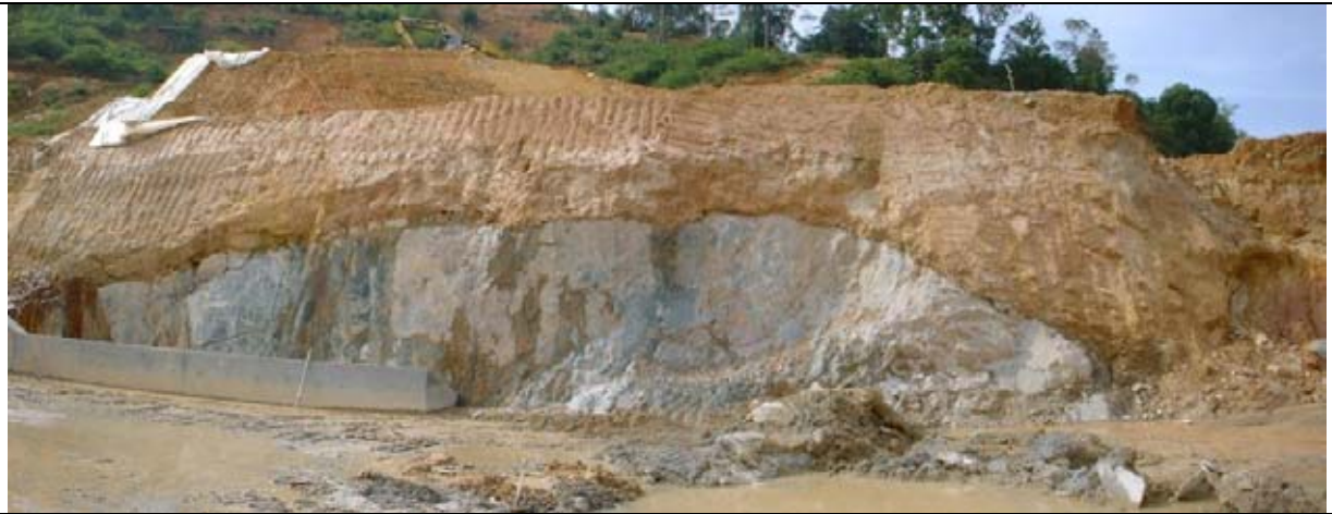
Figure 9 : Inconsistent Weathering
