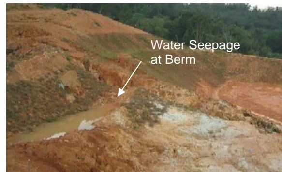
Figure 4 Water Seepage at Berm
