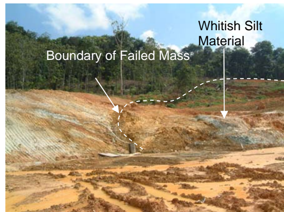
Figure 2 Front View of Failed Slope
