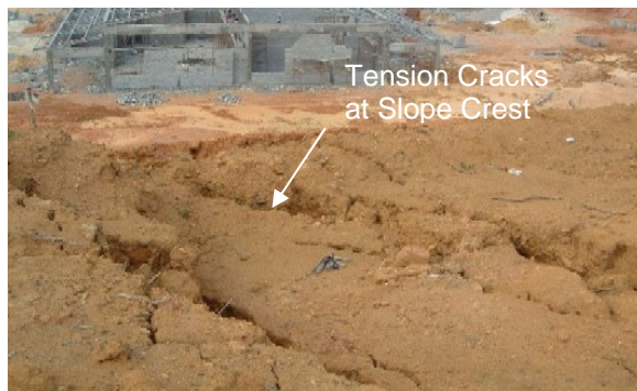
Figure 3 Tension Cracks at Top of Slope
