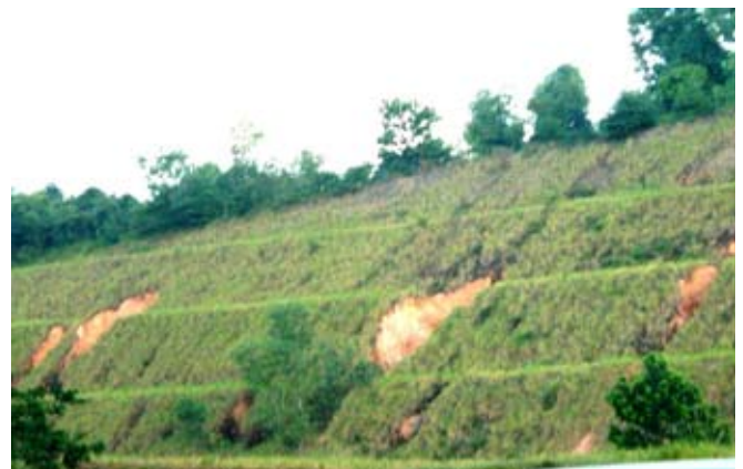
Figure 12: Localised Erosion on Slopes
