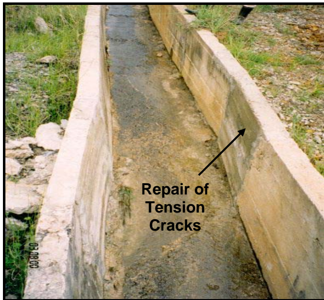
Photo 7: Repaired Cracked Drain
