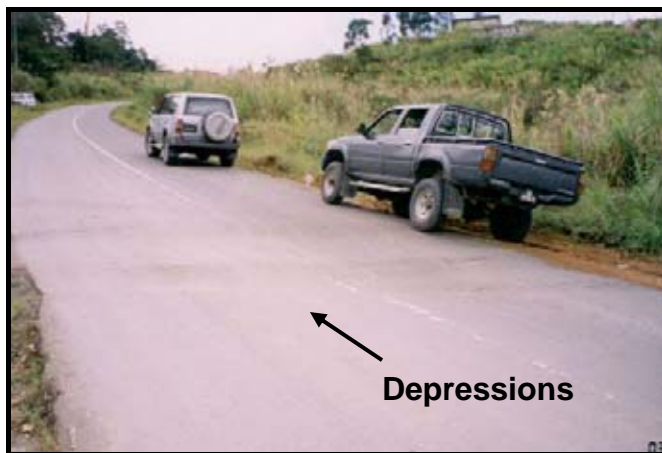
Photo 8: Depression on Road Pavement
