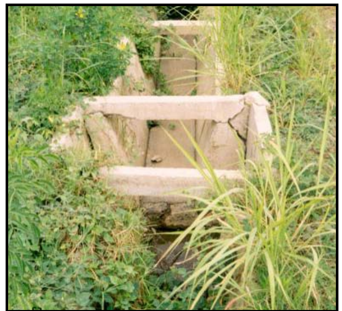
Photo 6: Distorted Drain Sump
