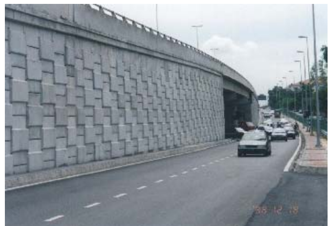
Photo 1: Side View of the RE Wall Embankment
