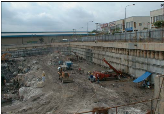
Photo 1: The Retaining System; Contiguous Bored Piled Walls (CBP) and Jack-in Soil Nails
